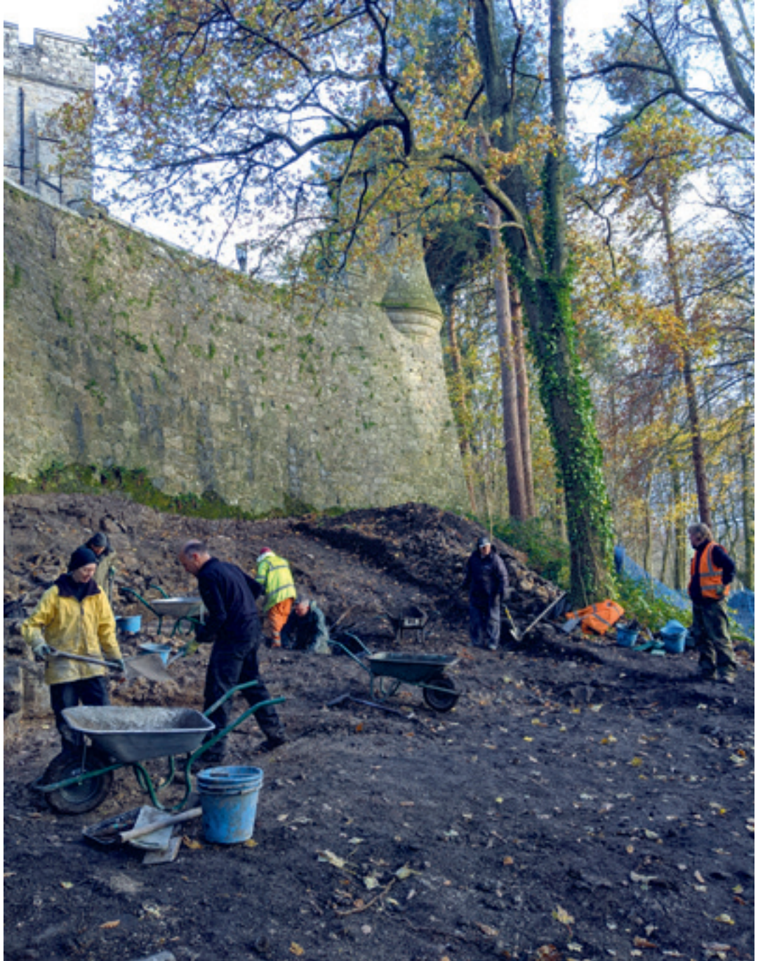
Working in a bubble or in their own, socially distanced spot – volunteers found plenty of space in the trench. © CPAT
