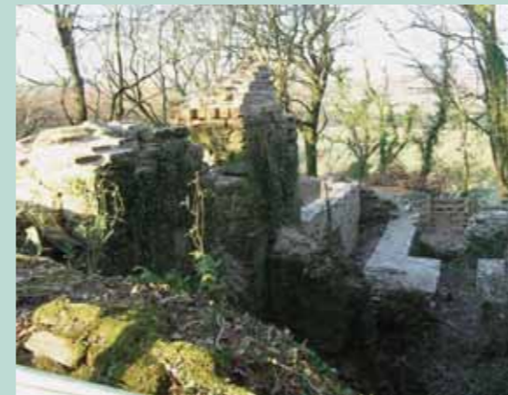
Wheal Tom (Deer Park Farm, Luccett, Cornwall). Remains of Wheal Tom Engine House, where all features were conserved using traditional methods and lime mortar. Site works included conservation of an arsenic chimney. Photograph: Colin Buck © Cornwall Council
