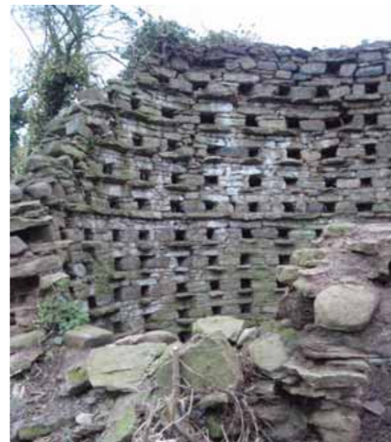
Thonglands medieval dovecote: Work in progress. Stone-by-stone recording preceded limited dismantling and reconstruction to secure the vulnerable fabric. © Mike Garner, Garner-Southall Partnership
