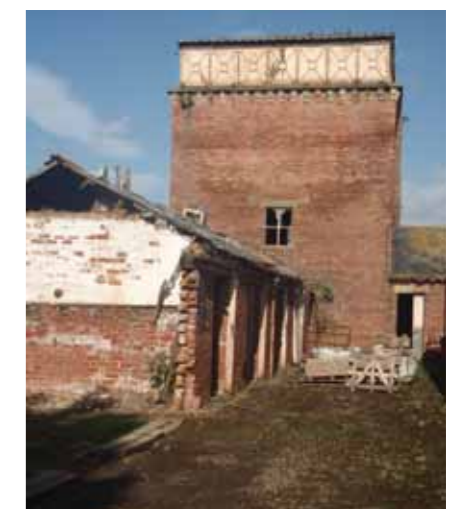
Myton on Swale, a Victorian model stud farm, built on an industrial scale in 1870, showing the ornate water tower and adjacent stable range
