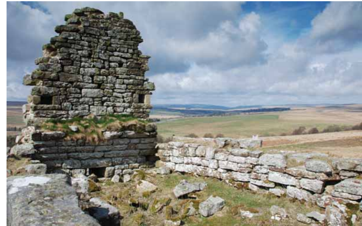
Shittleheugh Bastle, Northumberland, after Stewardship-funded work was complete
