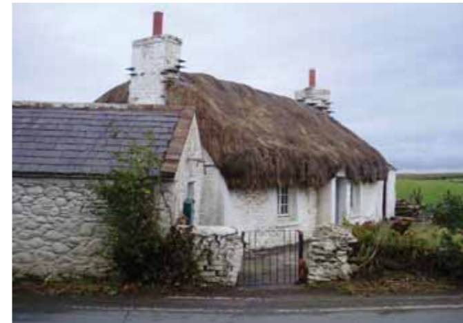
Thatched cottage at Cranstal, currently being restored with advice from the Manx Building Conservation Officer and the author. Recording of the building works has proved that the building is earthen-walled, behind facades of local brick
