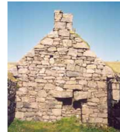
An internal gable of Pabbay House before consolidation and reapplication of eroded lime pointing
