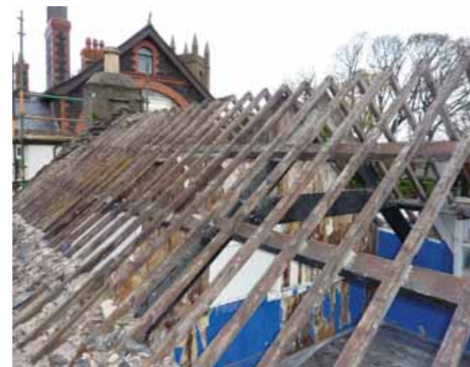
Rehanging the original slates on this early 19th-century cottage in Kirk Michael revealed a carefully made roof whose precision carpentry belies its low status. Note the vertically boarded timber partitions in the upstairs rooms
