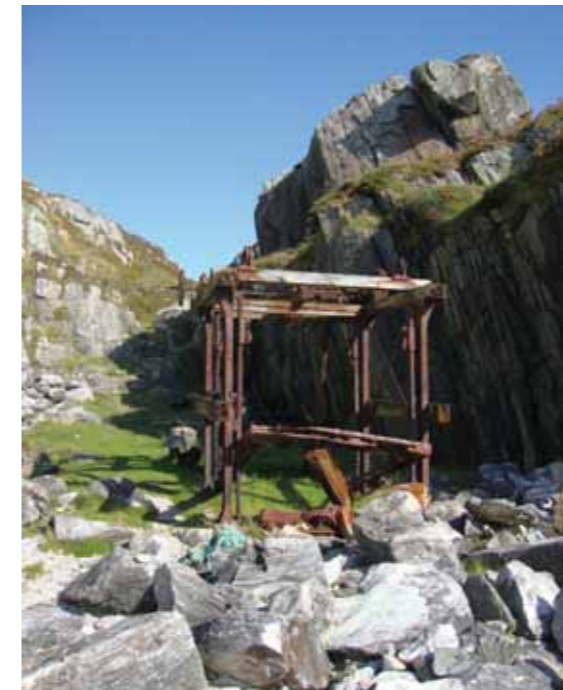
One isolated bay contains white marble that was briefly exploited. Equipment left behind when the quarry fell out of use at the onset of the First World War has recently been conserved by the National Trust for Scotland. Photograph: Alison Taylor
