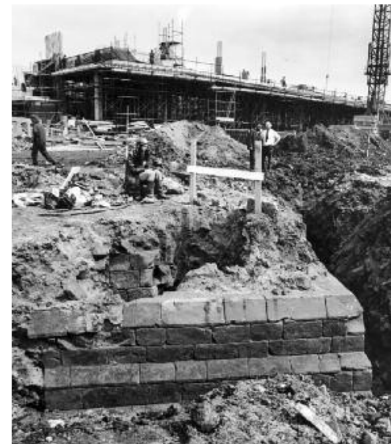
Stone wall exposed during construction of the Wholesale Markets on the manor house site. © Birmingham City Council
