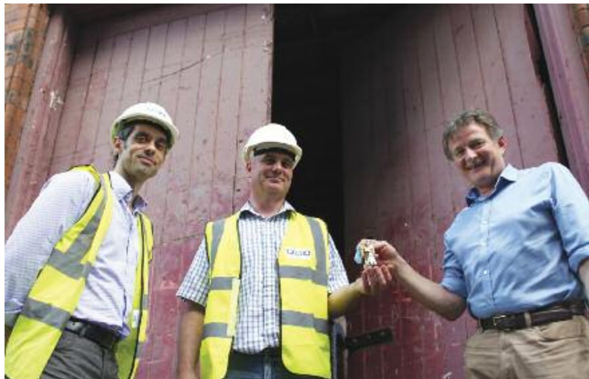
On 29 July the keys to the Coffin Works were finally handed over to contractors FWA, who are carrying out the repair and conservation work. From left to right: Ian Bird, FWA Contracts Manager, Andy King, FWA Site Manager, Simon Buteux, Director, Birmingham Conservation Trust. © Birmingham Conservation Trust
