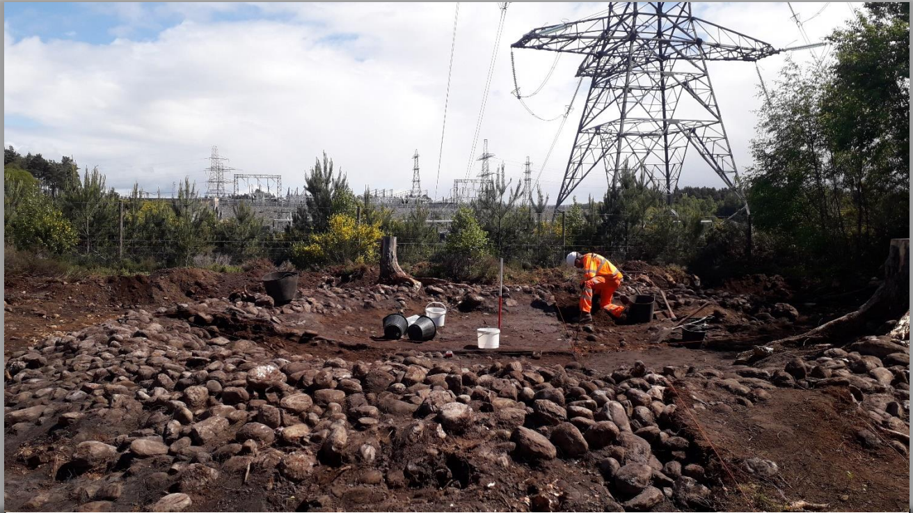
Excavations were part of a site survey for a new extension to the existing Beaully substation
