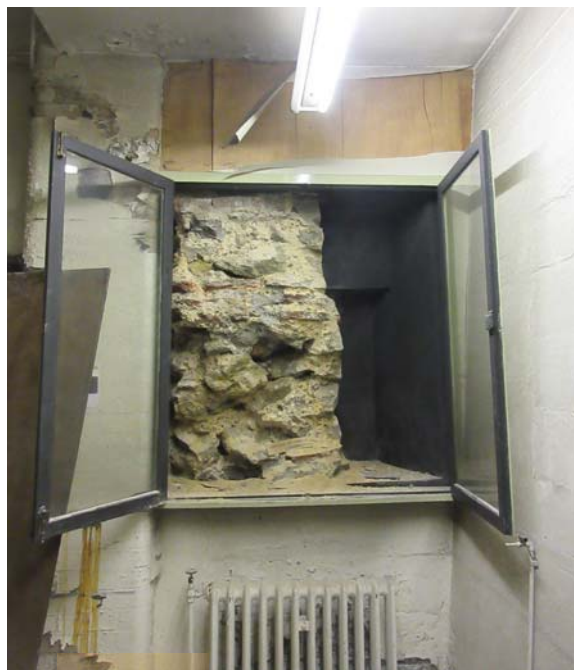
Designated remains of London City Wall, basement of project we are overseeing, City of London. Credit: Archaeology Collective
