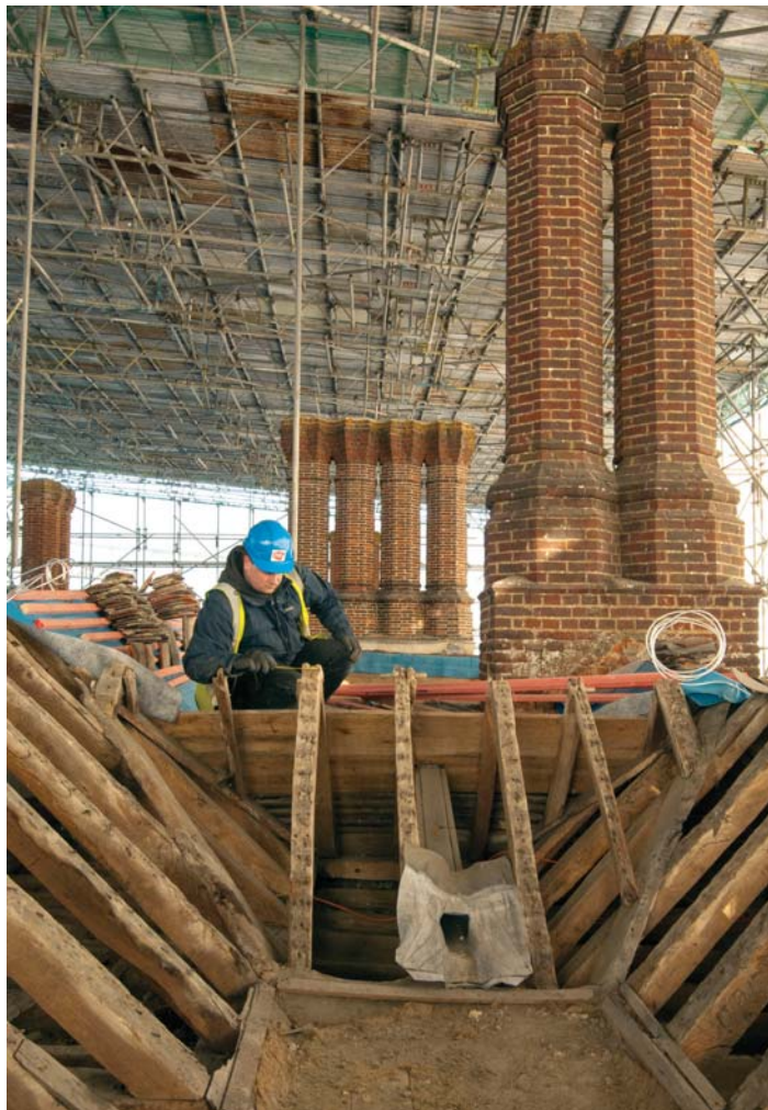
Knole House building recording. Credit: MOLA
