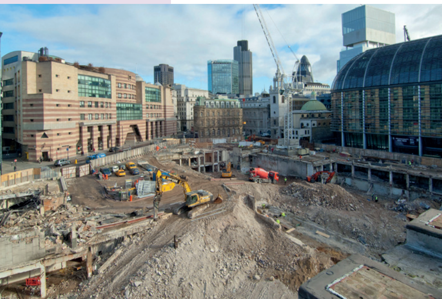
Bloomberg construction site during demolition (Photo: MOLA)
