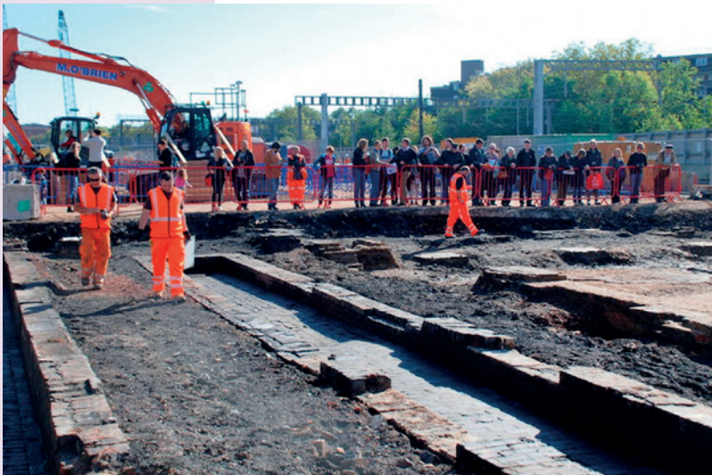
Open day at Westbourne Park (Photo: Jay Carver)
