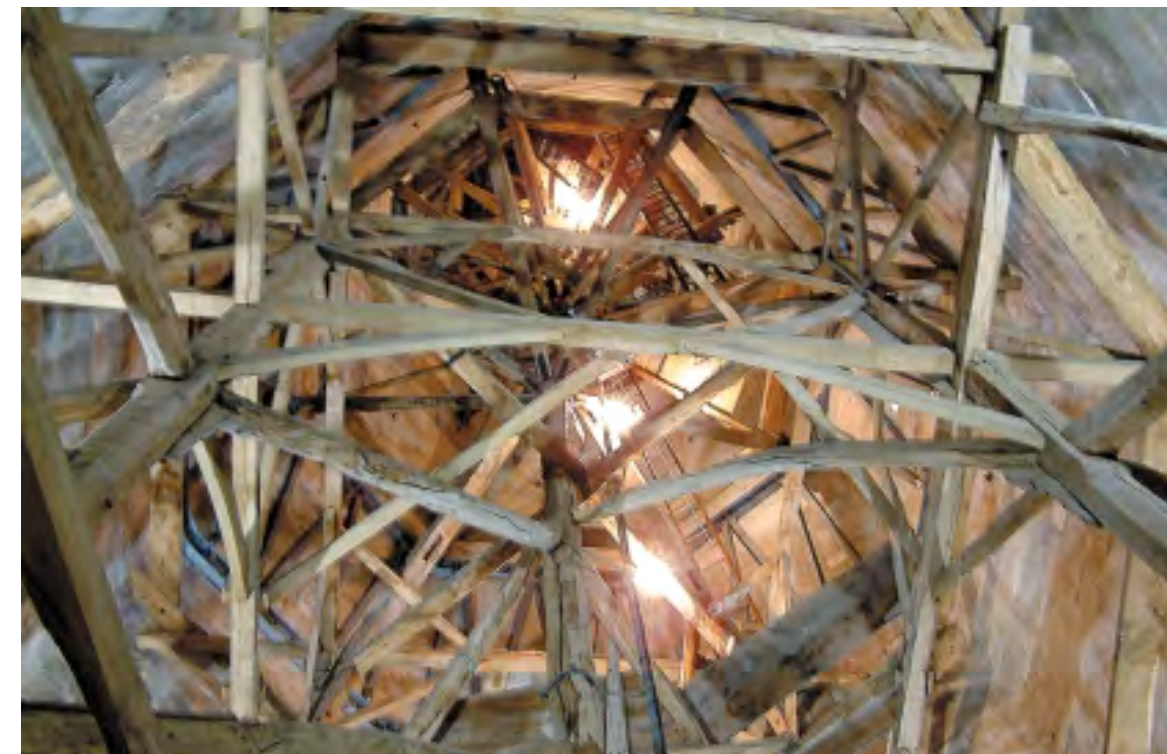
Interior medieval scaffolding within the Salisbury Cathedral spire from below. Photograph: Peter Marshall
