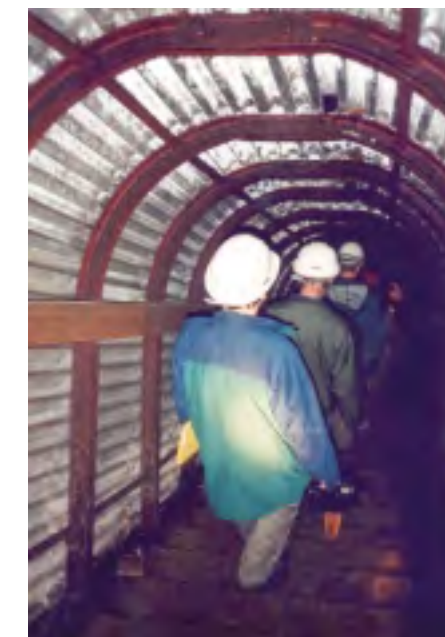
HMS Forward, Newhaven. Second World War Tunnels. Ensure you are equipped and prepared before you enter. © Paul Jeffery
