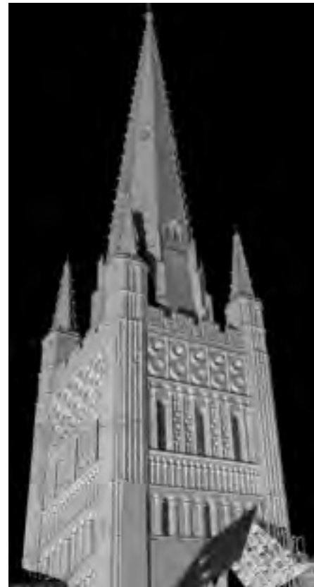
A point-cloud of Norwich Cathedral tower & spire; the results of a laser scan by APR Services
