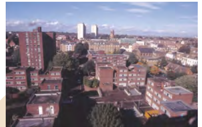
Acton: red-brick development of the 1970s, laid out around cul de sacs and predominantly low rise. Photograph: Derek Kendall © English Heritage
