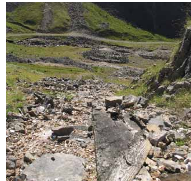
The crushing mill in the valley floor. In the foreground are remains of a timber chute which would have brought ore from the mines to the mill. © English Heritage
