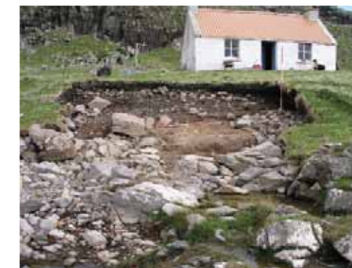
January 2005 storms. The massive bite taken out of the foreshore and the exposed foundations many metres behind the foreshore. The cottage was filled with beach gravel after the front door was smashed open
