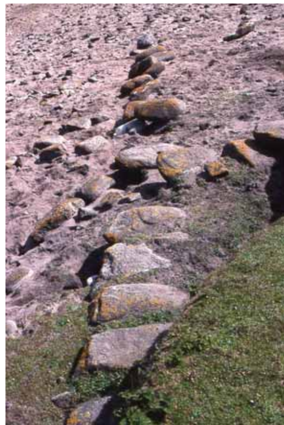
Structural elements being washed out and away at the Sheader site, Sandray 1995
