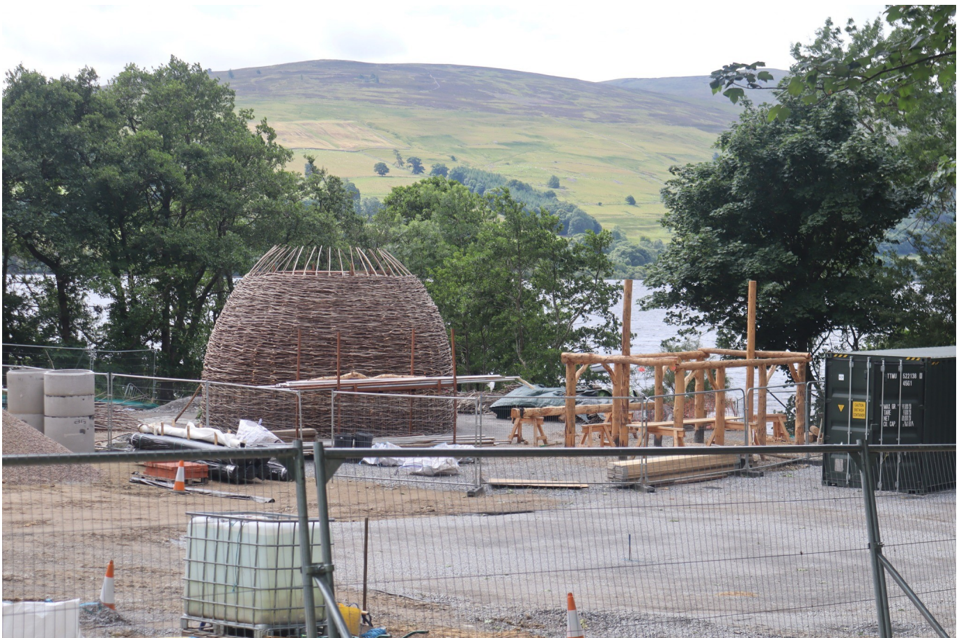
Image 1: A view of the progress of the roundhouse © Scottish Crannog Centre
