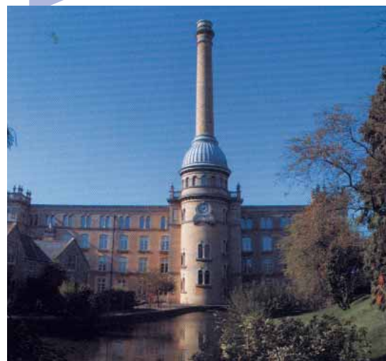
Residential conversion of Bliss's Tweed Mill, Chipping Norton, Oxfordshire
