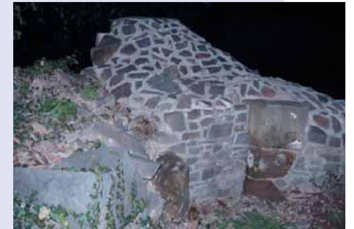
A filled-in cell in the north-east wall
