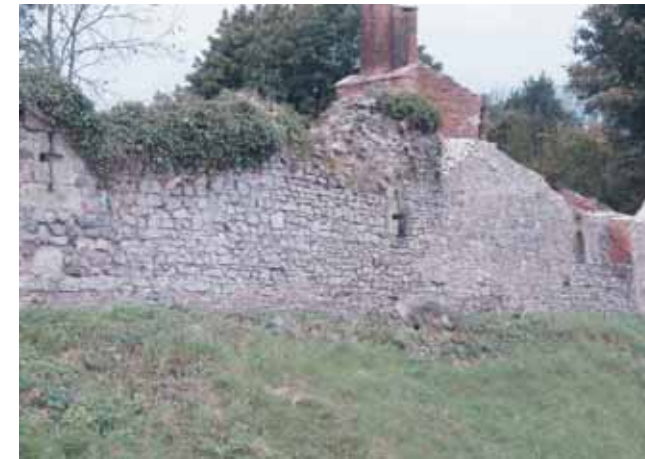
Hartshill east curtain wall
