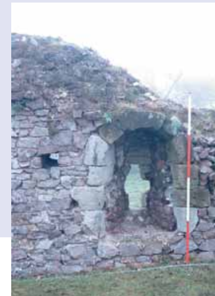
An embrasure in the south curtain wall
