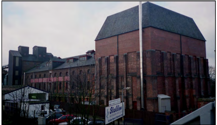
The south and east elevations of Beeston Maltings, taken in 2000 just before closure. Credit: Amber Patrick.
