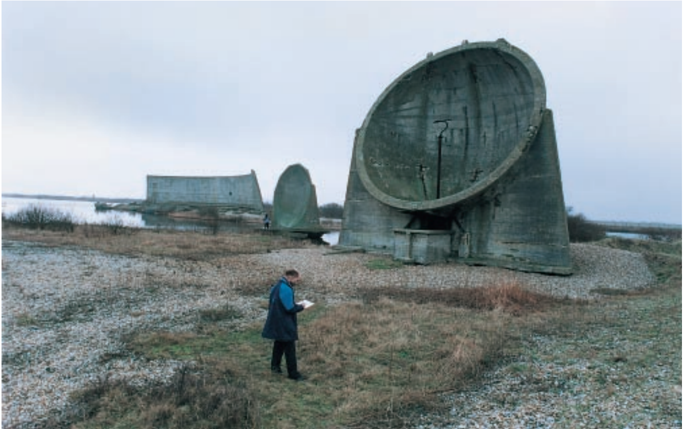
Recording underway as part of the Defence of Britain project. The 1928 pre-radar sound mirrors at Denge, Kent, are inspected by the Volunteer Coordinator for the south of England. Photograph David Mansell
