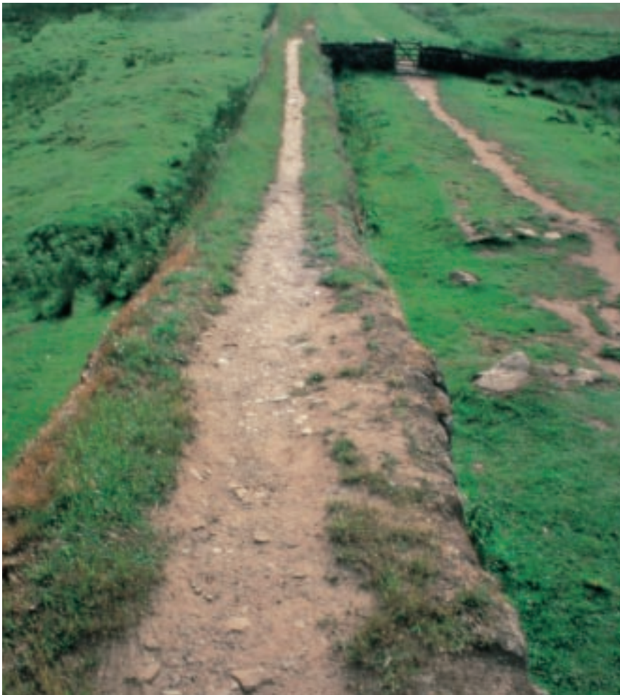
Hadrian's Wall near Steel Rigg, showing erosion caused by walkers on the wall. Two major awards from HLF, totalling more than £3 million, have helped the Countryside Agency establish the Hadrian's Wall path, which will provide access to the Wall from end to end, but also ensure that the impact of visitors on the wall and its surroundings will be managed. Photograph HLF Photographic Library
