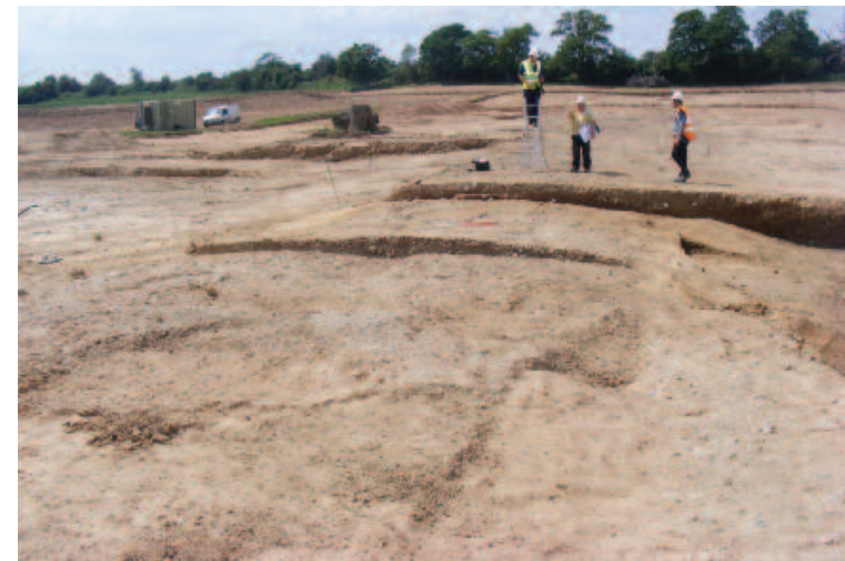
A general view of the site showing three phases of road construction © SLR Consulting
