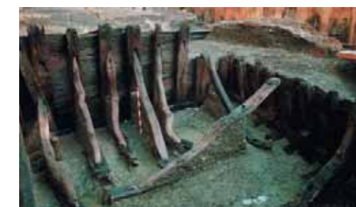
Billingsgate Saxon revetments in situ. These will be part of the new displays. Photograph: Andy Chopping
