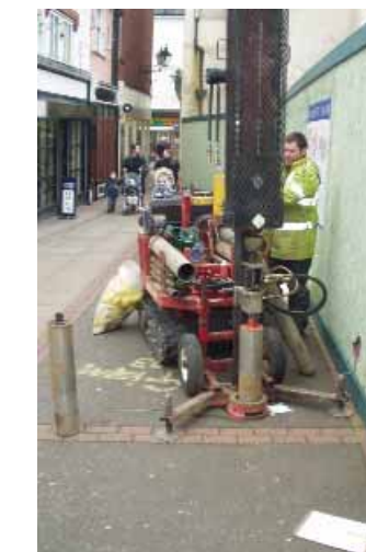
Coring in Market Row. Photograph: Ken Hamilton
