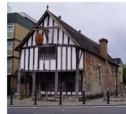
58 French Street, a medieval merchant's house, adjacent to the site. © Oxford Archaeology
