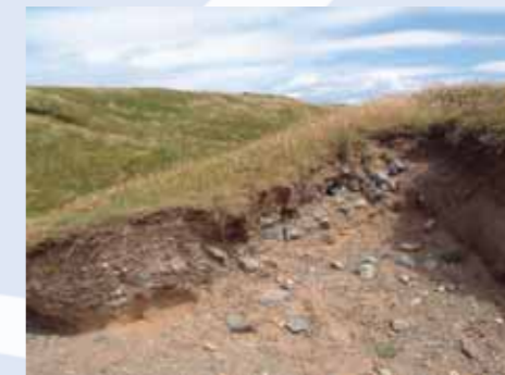
Internal construction details in part of a rampart eroded by the footpath
