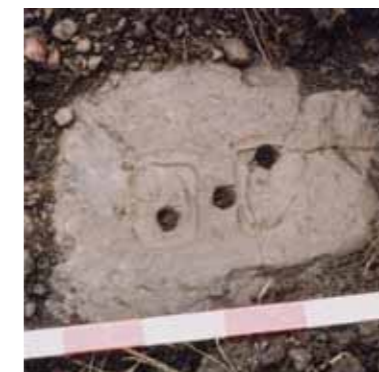
Type B sleeper block showing the impression of the feet of the iron chair. The hole in the middle indicates it may be reused from a type A block that has been turned over
