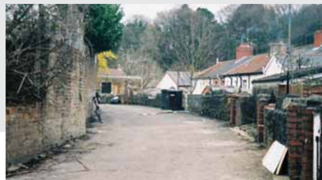
The line of the tramroad preserved along a back road of terraces in Merthyr Tydfil
