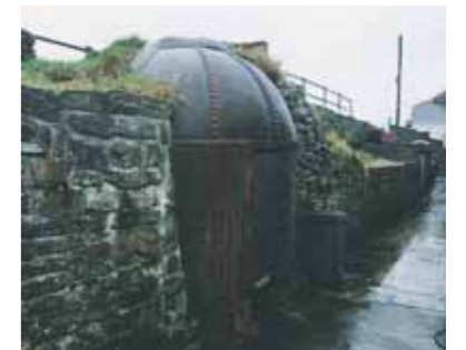
Abercanaid haystack boiler, Merthyr Tydfil. The boiler is a rare and early example of steam engine technology. It is believed to have been used at the Gethin Pit and brought down to Abercanaid in the 1930s, where it was used as an air raid shelter during the Second World War. © Cadw, Welsh Assembly Government (Crown Copyright)
