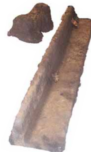
Tramplate and 'Type B' chair, showing the L-shaped section
