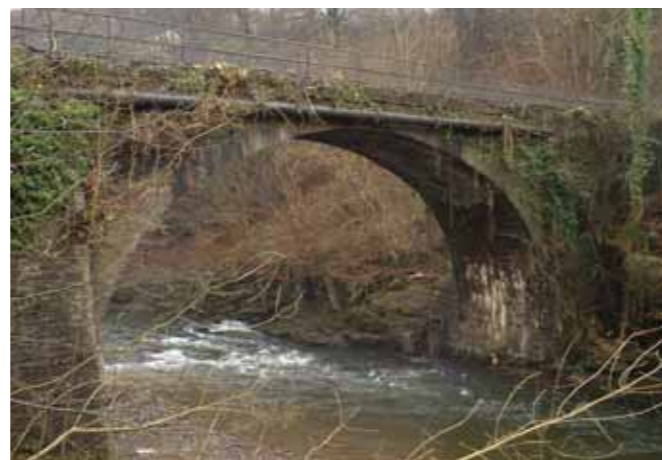
Quaker's Yard tramroad bridge
