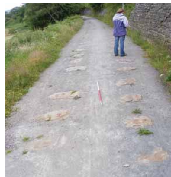
Type B sleeper block showing the impression of the feet of the iron chair. The hole in the middle indicates it may be reused from a type A block that has been turned over
