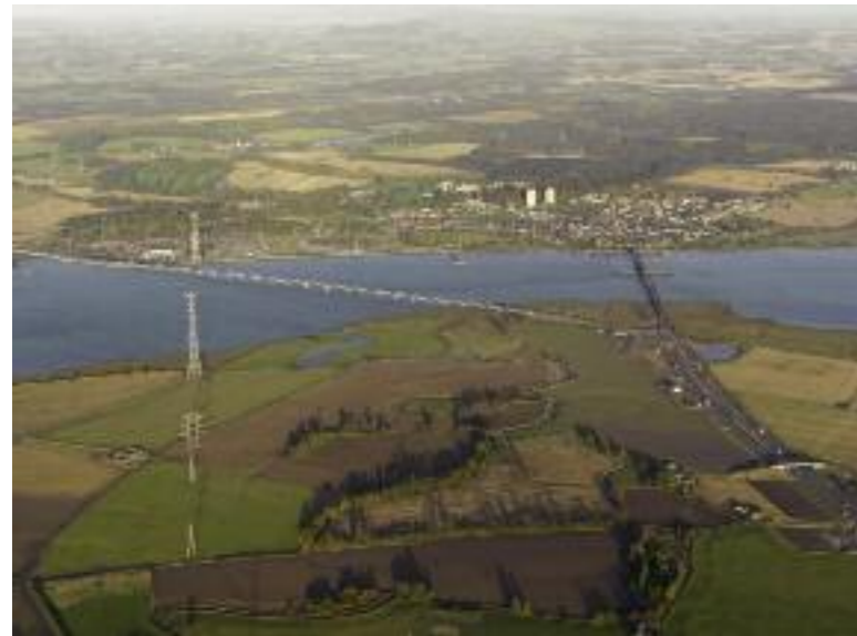
A876 Upper Forth Crossing: recently completed after a developer-funded programme of archaeological investigation ranging from Neolithic settlement (close to the nearer shore) to the 19th century. Note the A-listed Kincardine Bridge to right of shot © Transport Scotland
