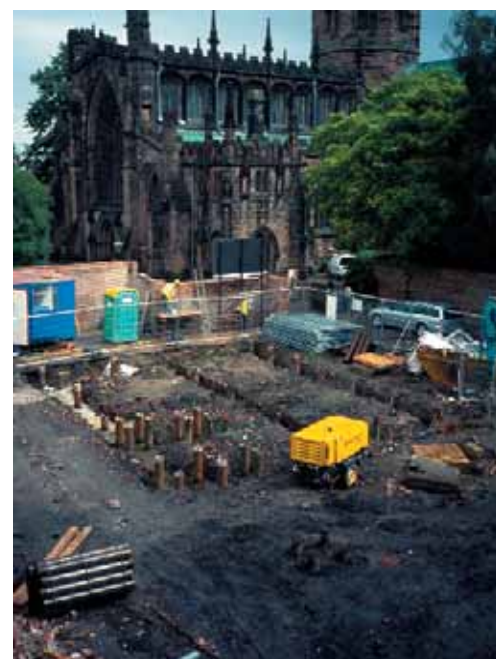
Excavations at the Lamb Hotel with remains of Anglo-Norman timber structures, and piling in progress © Gifford
