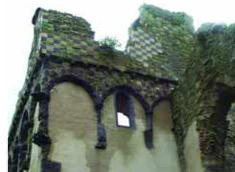
A decorative arcade parapet runs around the top of the main ranges displaying a colourful chequerboard design comprised of purple Caerbwdy sandstone, cream-coloured limestone and white quartz. Selective restoration undertaken as a conservation measure also enables visitors to appreciate the overall decorative design
