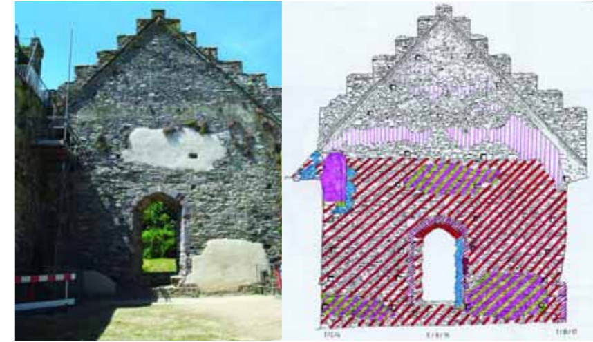
A typical work specification drawing and the finished wall. Note the new render which protects an area of vulnerable Porthlysgi volcanic tuffs. The fresh white colour will fade over time
