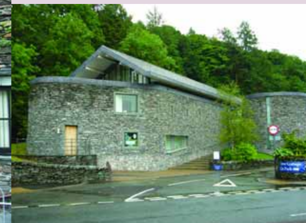
Evidence that conservation area status need not stifle bold modern design: the Wordsworth Centre in Grasmere Town End
