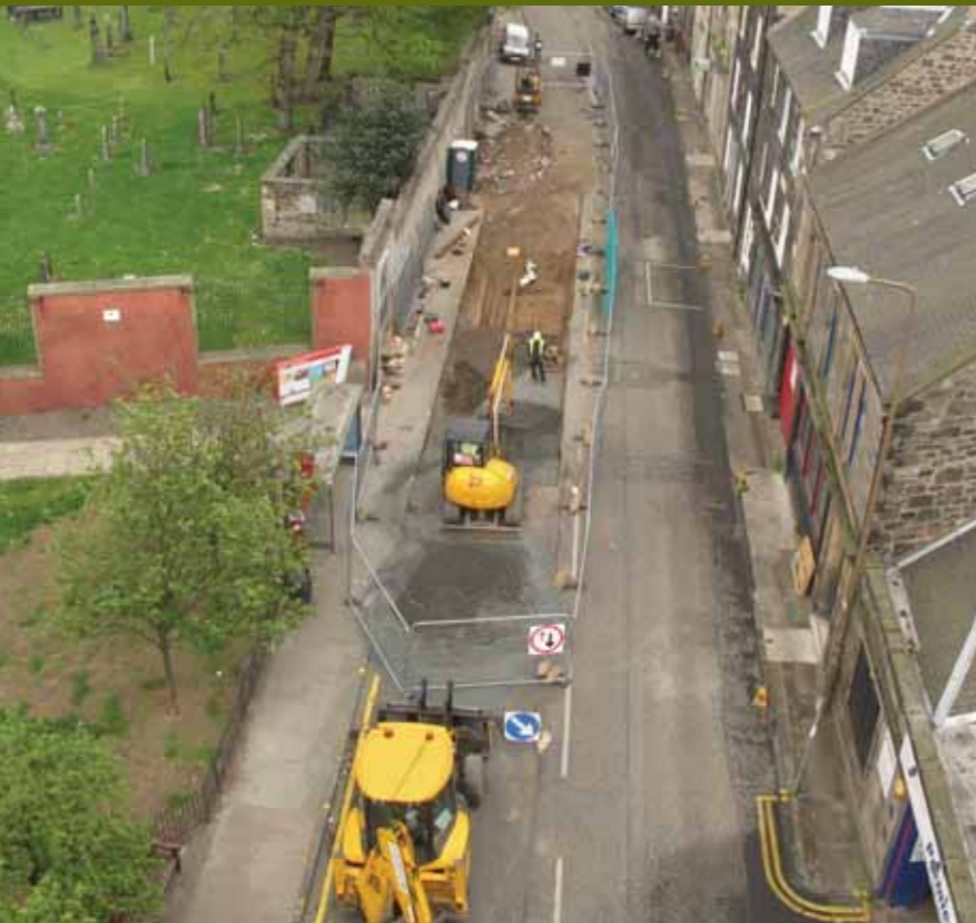
Constitution Street looking north, with the graveyard and wall to the west
