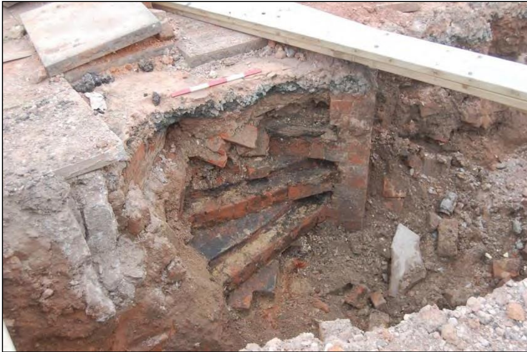
Fig 19: Spiral brick staircase (formerly with timber tread-nosings) down to a Parkside cellar, looking south; scale 0.5m
