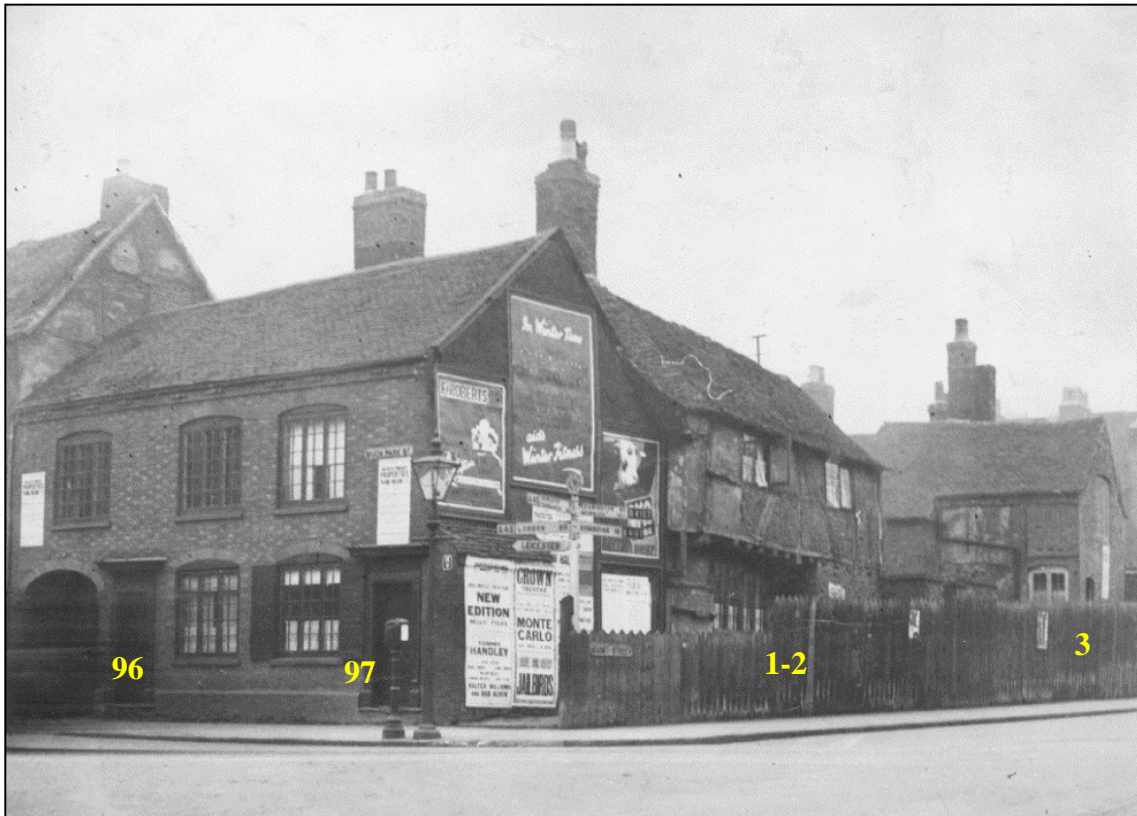
Fig 2: A photograph taken between 1900 and 1931 looking south and showing nos 96-7 Much Park St, with nos 1-3 Short Street (separated rear wing and converted former outbuildings) behind. The rear wing of no 97 (1-2 Short St) is clearly timber-framed, jettied out and brick-nogged, being perhaps of 15 th -17 th century date. The frontage of nos 96-97 show all the brickwork and window/doorcase shapes typical of the late 18 th - to early 19 th century and an arrow-straight ridge-line, hardly the stuff of slums awaiting clearance. The gable end of the 1711 Three Swans Inn (Nos 94-5) is at far left, apparently box-framed with brick-nogging. At far right is 3 Short Street, which stood over an excavated basement room. It appears to be of brick, probably itself a re-build.
