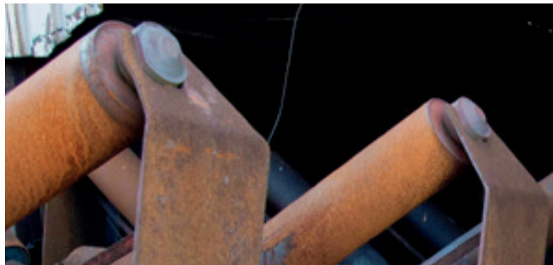
Blast Furnace detail ©TEP
