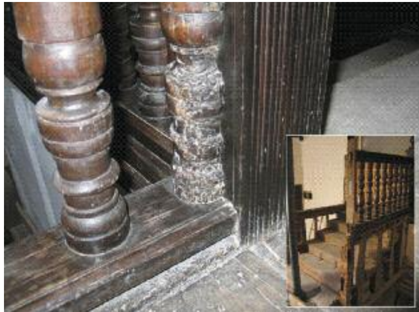
Is this really the "good 17th C stair" the List description would have us believe? (Mike Heaton)
