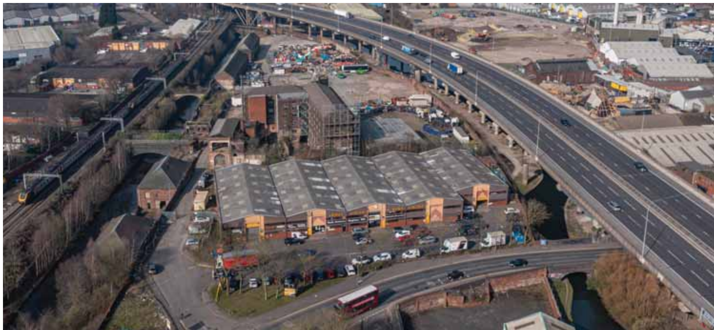
A view of the site today. Nestled between the M5, railway and canals, the seven-storey structure (seen here with scaffolding) and canal side buildings formed part of the extensive glass works. Credit: Aerial-Cam
