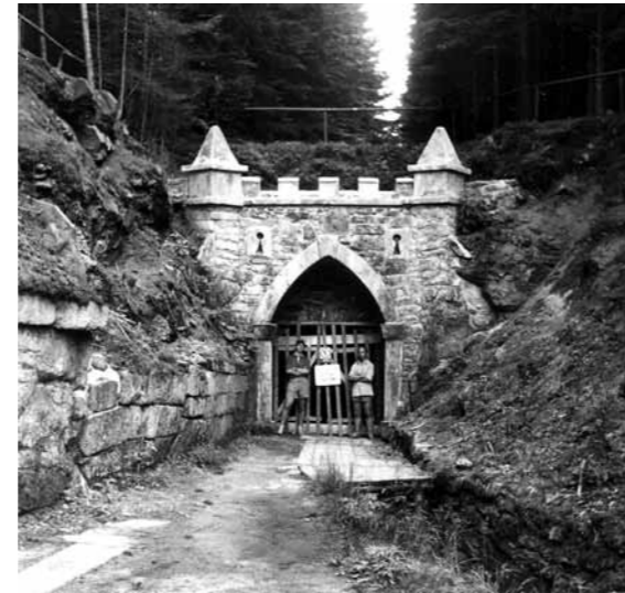
An elaborate portal of the Schwarzenberg logging sluice tunnel. 419m long and dated 1823
