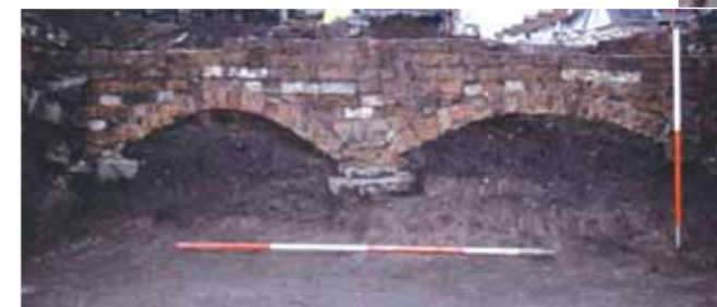
Arched foundations of the terraced houses. Photograph: D Gilbert (JMHS)
