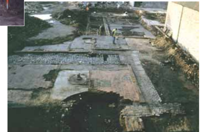
Recording in progress of 19th-century industrial buildings. Photograph: D Gilbert (JMHS)
