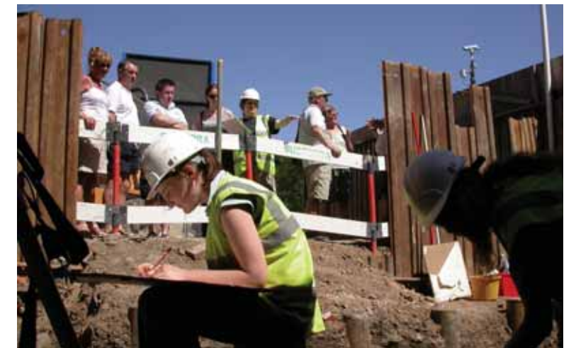
Visitors to Bedford High Street are drawn into more understanding of their historic environment by direct engagement with work in progress
