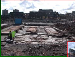
Trent Sanitary Works, Hanley
