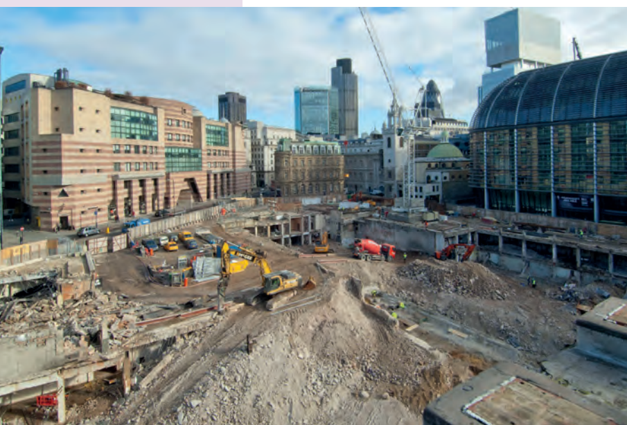
Bloomberg construction site during demolition (Photo: MOLA)
