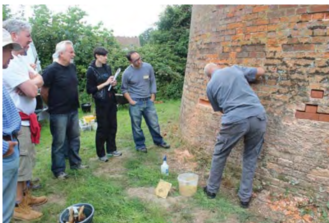
An Introduction to Traditional Brickwork Repairs for Beginners: Stock Windmill. Credit: Place Services
