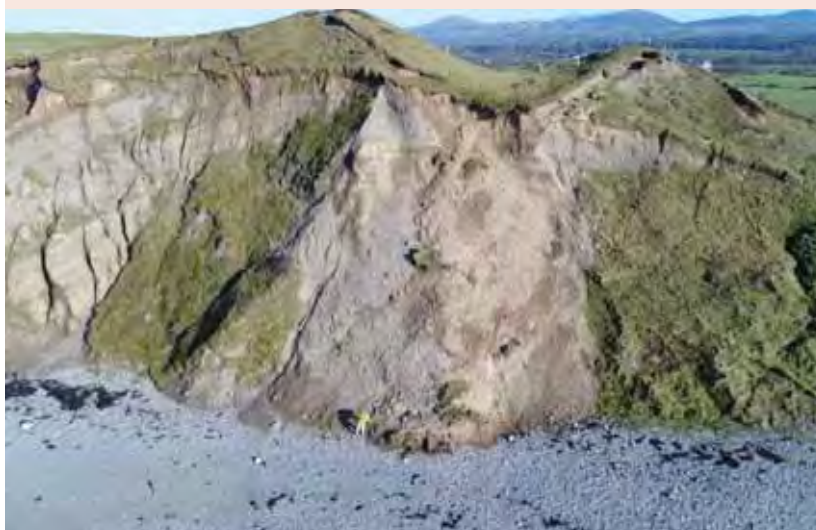
Fresh cliff collapse below the southern hillfort ditch, recorded on 14 Feb 2019, was exacerbated by intense rainfall funnelling water along the fort's ditch. Crown Copyright: CHERISH Project 2019
