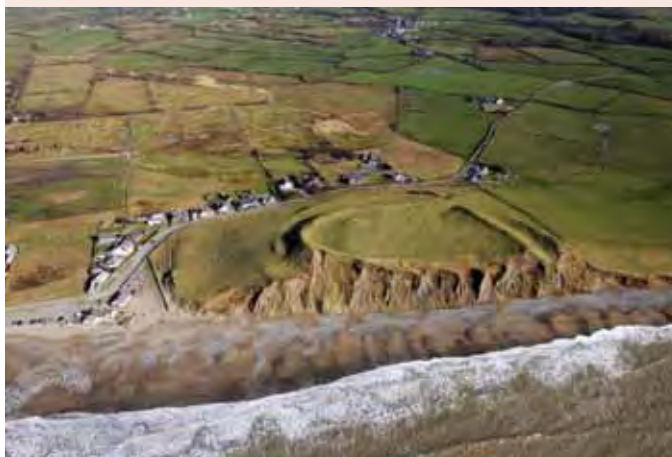
Dinas Dinlle is owned by the National Trust. It is protected as a Scheduled Monument whilst the cliff face itself is a Site of Special Scientific Interest, designated for the geological importance of exposed glacial sediments. Crown Copyright: RCAHMW AP_2014_0877
