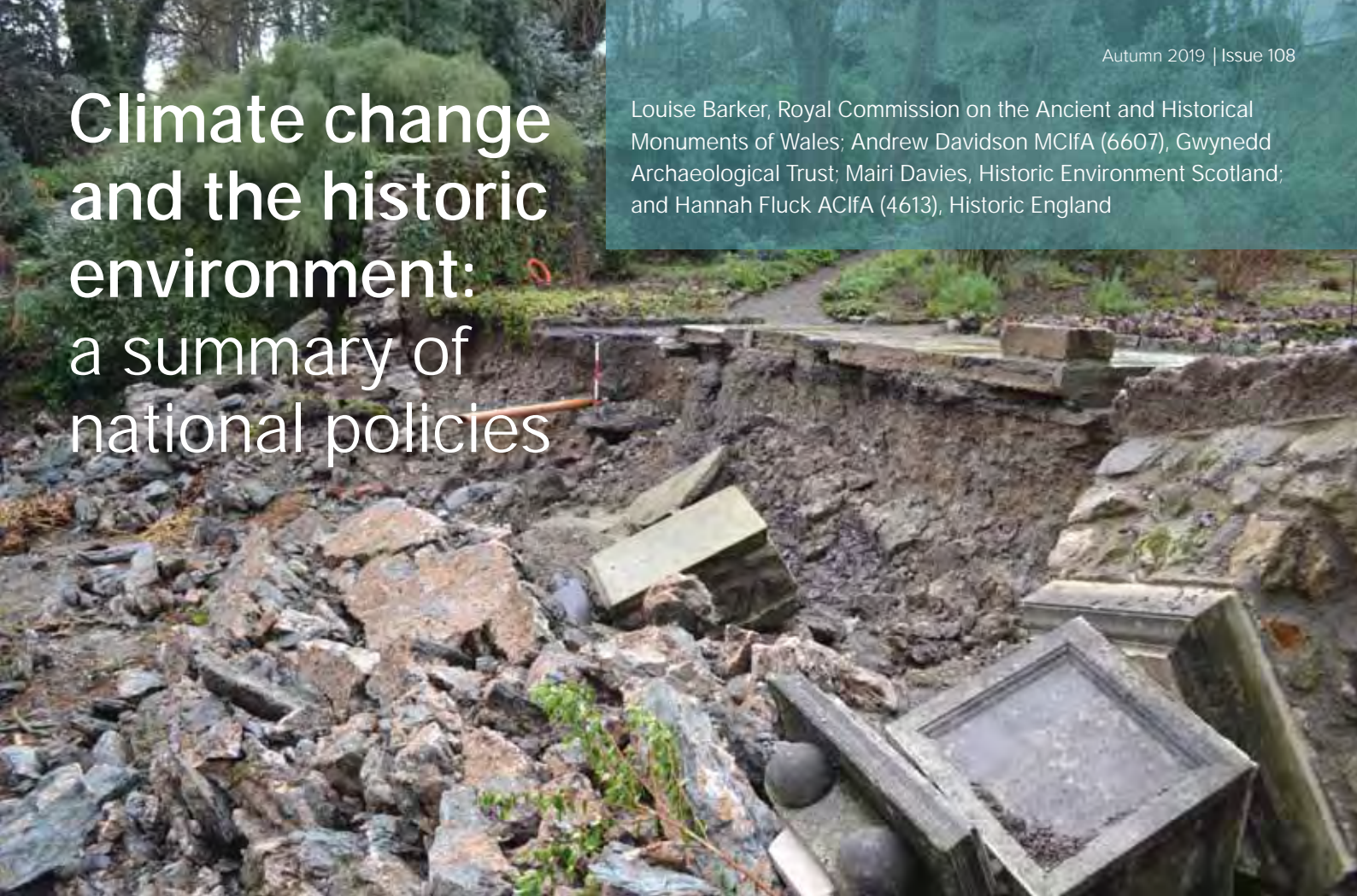
Damage at Plas Cadnant historic gardens, Anglesey, following excessive rainfall in 2017. Credit: Gwynedd Archaeological Trust
