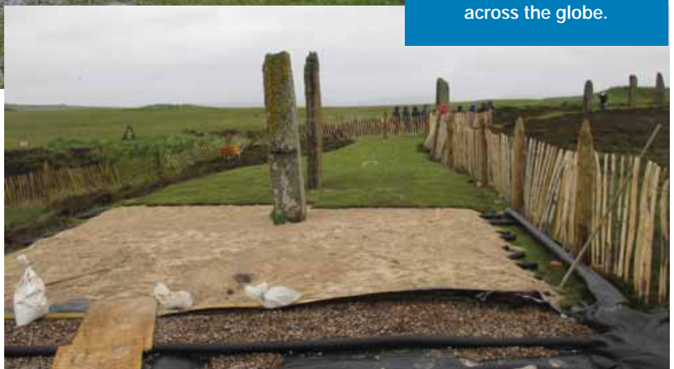
(right) Installation of engineered surfaces to improve footpath resilience at the Ring of Brodgar. Credit: Historic Environment Scotland
