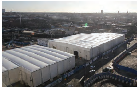
Bird’s-eye view of excavation tents looking south west. Credit: LMJV
