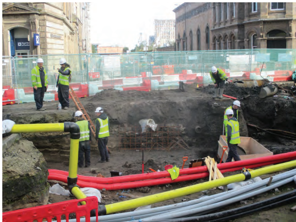
Archaeologists often encounter underground infrastructure during fieldwork: Edinburgh Tram Extension 2020, GUARD Archaeology excavating the junction of Constitution St. and Baltic Street Junction, Leith. Credit: CECAS 2020
