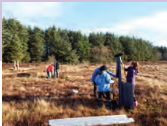
Ditch-blocking in process. Credit: Peatland ACTION project, NatureScot
