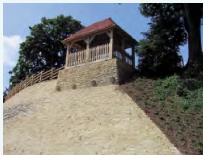
The ‘tower’ with new green oak shelter and rebuilt revetment wall
