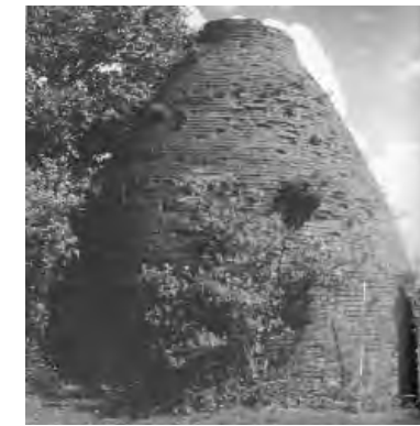
Brick-built bottle-shaped craft pottery kiln, c. 1830, at Sutton Coldfield
