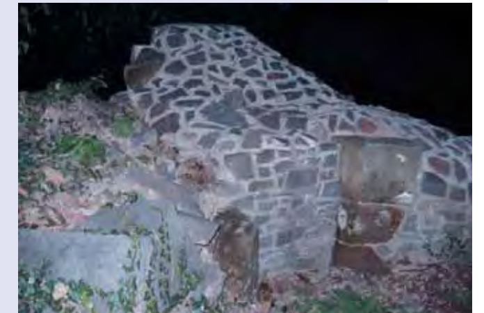
A filled-in cell in the north-east wall
