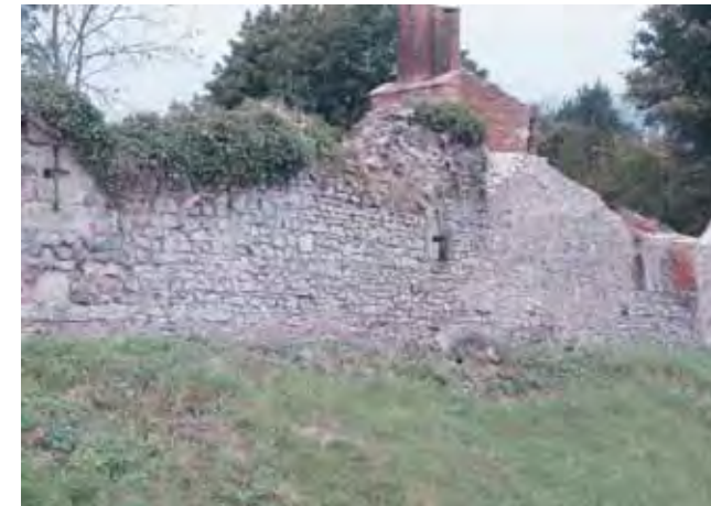
Hartshill east curtain wall
