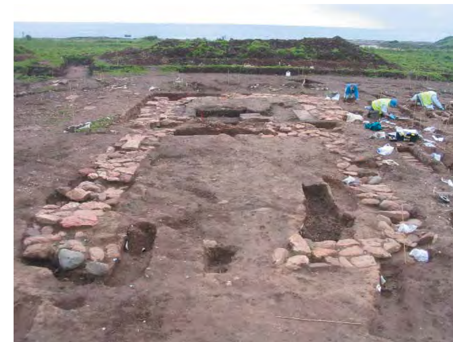
Foundations of the chapel. The earliest building lies in the foreground with a more substantial later addition beyond. Bamboo canes mark burials.
