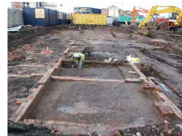
The Greengate Towers development, partly excavated by Oxford Archaeology North in 2006, showing a row of cellared dwellings. The back yards lay over a deep black garden soil which yielded a substantial assemblage of 17th/18th century pottery. A 13/14th century boundary ditch runs across the top of the excavation area
