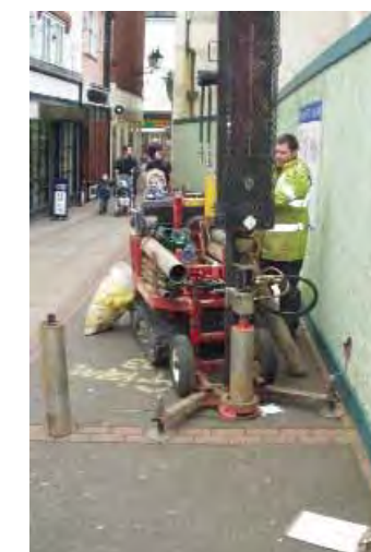
Coring in Market Row. Photograph: Ken Hamilton
