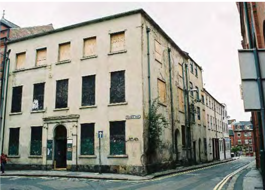
41 Pilcher Gate, Nottingham – proposed for demolition. Photograph: the Georgian Group
