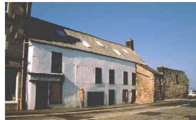
Dymock's Building: north façade, before restoration. © NTS
