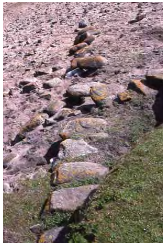
Structural elements being washed out and away at the Sheader site, Sandray 1995
