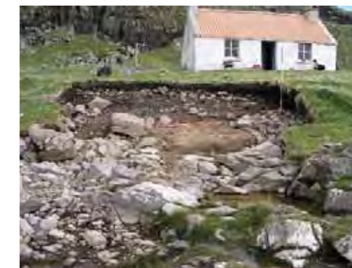
January 2005 storms. The massive bite taken out of the foreshore and the exposed foundations many metres behind the foreshore. The cottage was filled with beach gravel after the front door was smashed open
