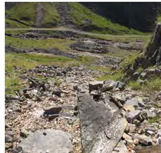
The crushing mill in the valley floor. In the foreground are remains of a timber chute which would have brought ore from the mines to the mill. © English Heritage
