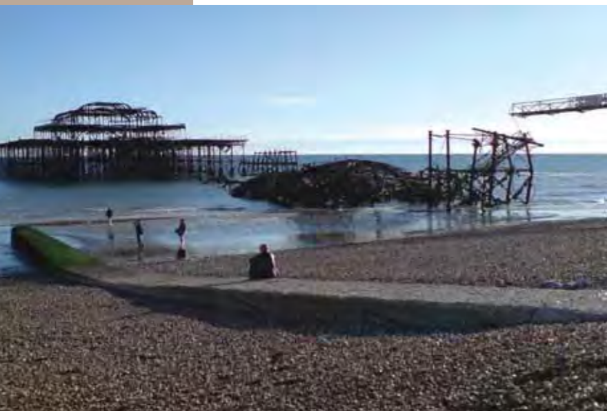
The West Pier at Brighton after its destruction. Photo: Kathryn Whittington
