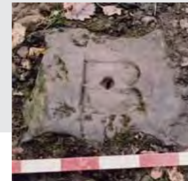
A Merthyr Type A sleeper block
