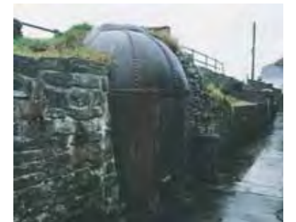
Abercanaid haystack boiler, Merthyr Tydfil. The boiler is a rare and early example of steam engine technology. It is believed to have been used at the Gethin Pit and brought down to Abercanaid in the 1930s, where it was used as an air raid shelter during the Second World War. © Cadw, Welsh Assembly Government (Crown Copyright)
