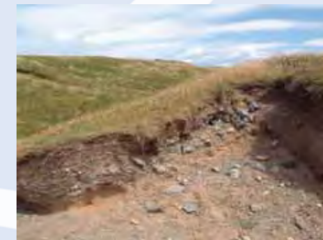
Internal construction details in part of a rampart eroded by the footpath
