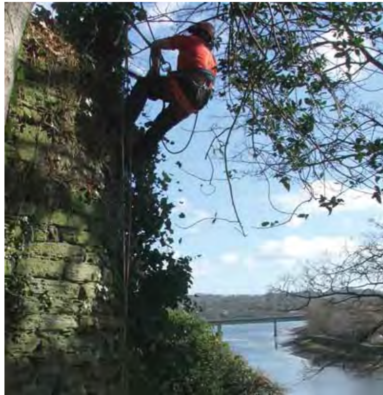
Removing vegetation on Cardigan Castle, before building recording. © Ceredigion County Council
