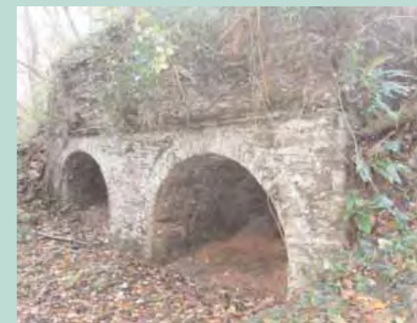
Rowlestone Limekiln Tunnels. These dual tunnels are built into the hillside and sit below the melting pot, which would have been layered with charcoal and limestone before heating
