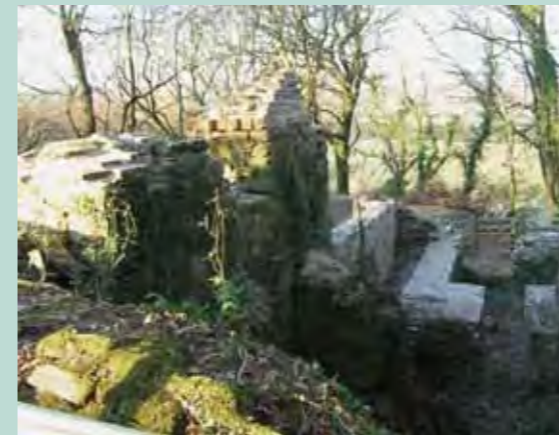
Wheal Tom (Deer Park Farm, Luccett, Cornwall). Remains of Wheal Tom Engine House, where all features were conserved using traditional methods and lime mortar. Site works included conservation of an arsenic chimney. Photograph: Colin Buck © Cornwall Council
