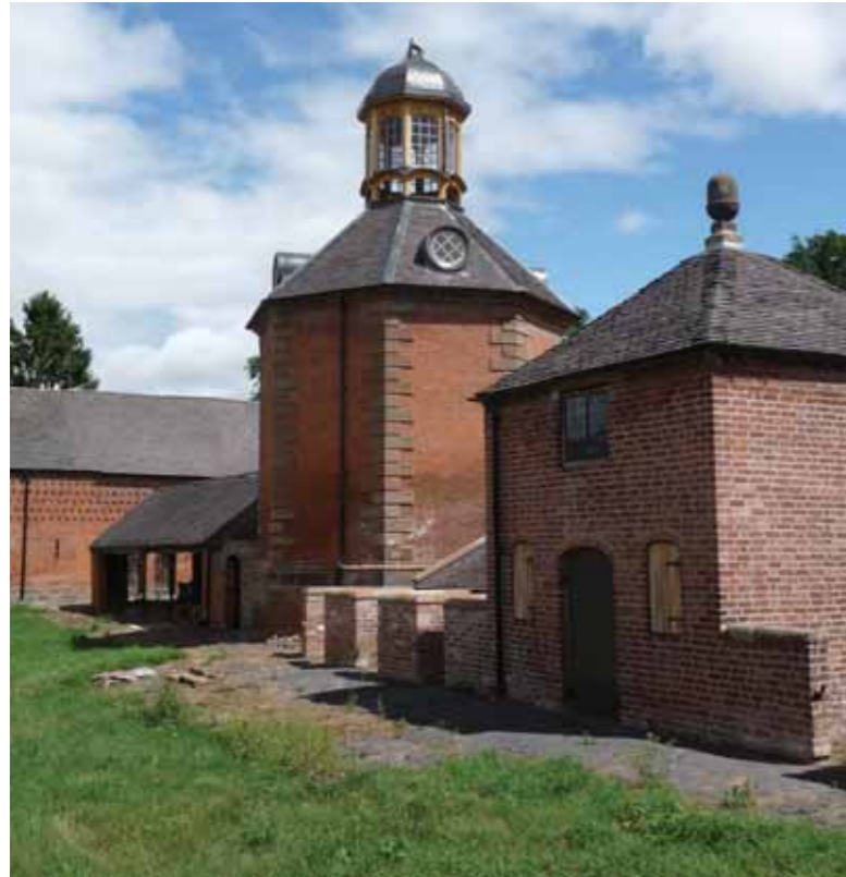
The dovecote at Chillington after conservation in 2010. Photograph: Horsley Huber Architects
