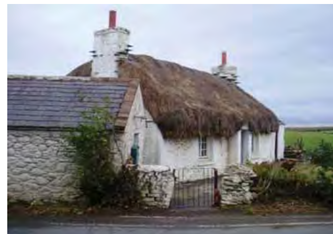
Thatched cottage at Cranstal, currently being restored with advice from the Manx Building Conservation Officer and the author. Recording of the building works has proved that the building is earthen-walled, behind facades of local brick
