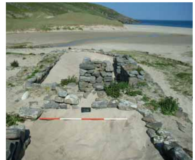
Monitoring blackhouse ruins: recording structure by structure the ingress of wind-blown sand and the location of rabbit burrows. © National Trust for Scotland
