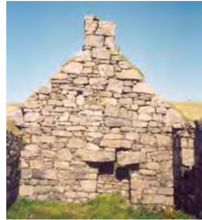
An internal gable of Pabbay House before consolidation and reapplication of eroded lime pointing
