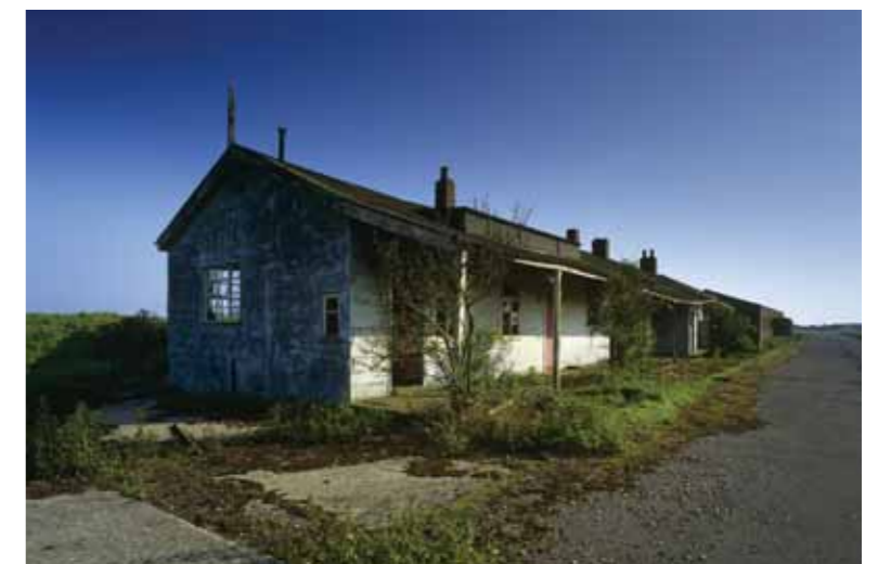
The 'Street' of derelict buildings on Orford Ness. ©NTPL/Joe Cornish
