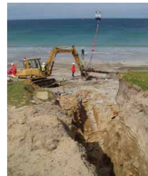
ORCA monitoring cable landfall at Skail Bay, Orkney © ORCA
