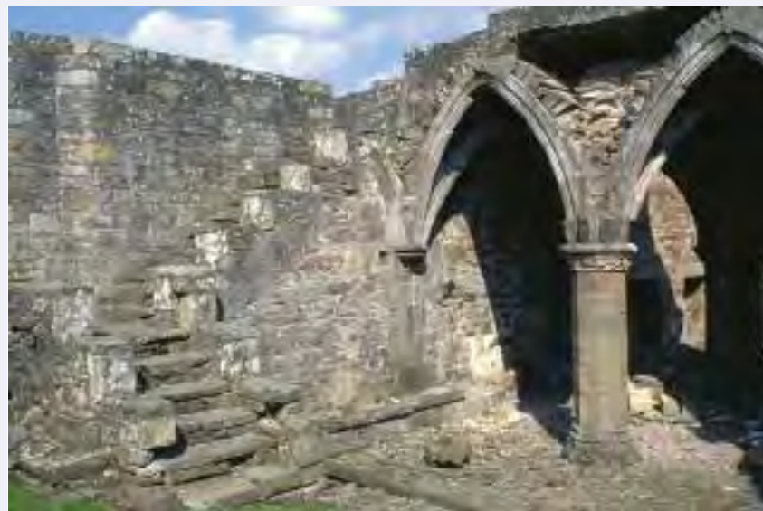
Photo of Balmerino Abbey – the Canmore record has received recent updates from both RCAHMS thanks to a special survey project and the National Trust, who recorded a watching brief as a result of the replacement of an interpretation panel. http://canmore.rcahms.gov.uk/en/site/31746 . Copyright: National Trust for Scotland
