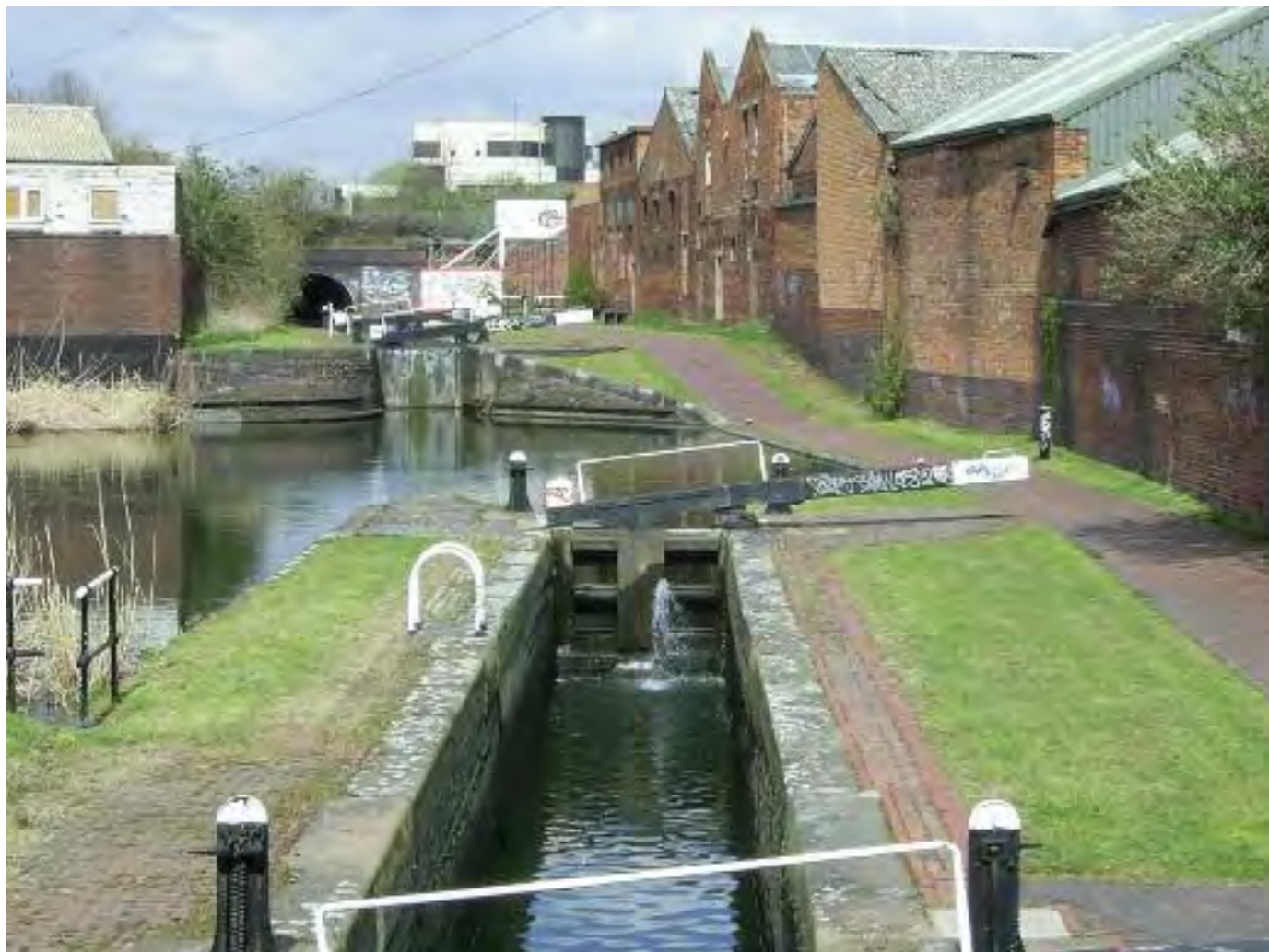
Ashted canalside and locks in the area of the Eastside Locks development. © Birmingham City Council
