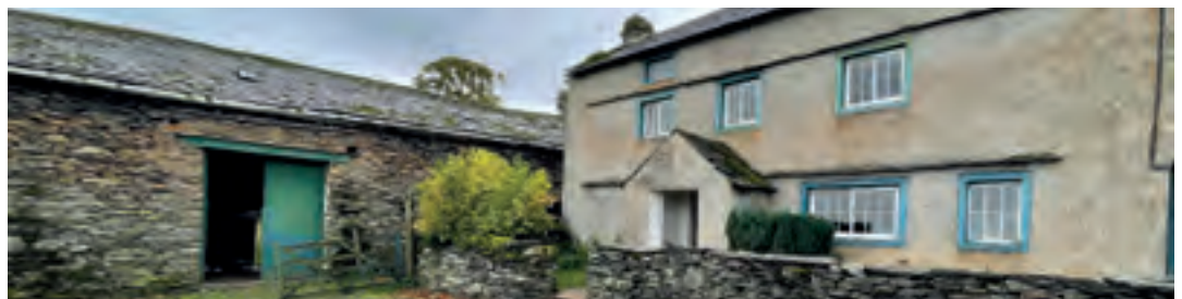
Eastward Farmhouse and attached barns, The Lake District
