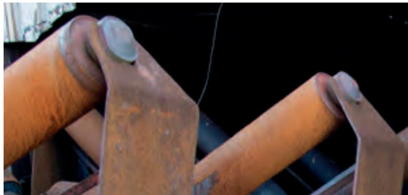
Blast Furnace detail ©TEP
