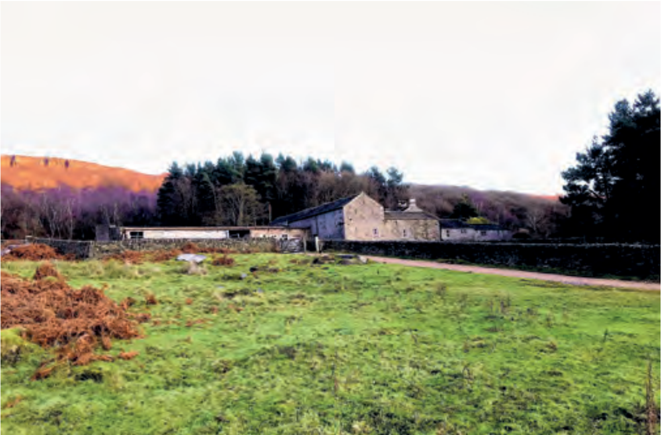
View of the farmstead from the west, showing the fragments of the early 20th-century shelter shed which has been retained as part of the scheme, and the main L-plan range to the right of the image. ©Jeremy Lake
