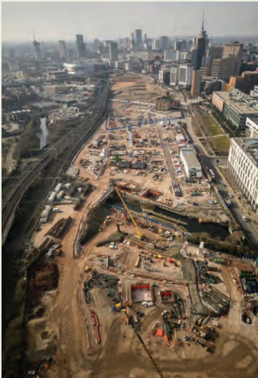
Aerial view of Birmingham High Speed Rail 2 construction. Credit: UAV 4 (Shutterstock)
